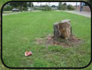
A stump could be dangerous for road users damage machines such as: Mowers, snow blades etc.
